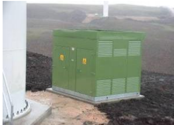
A bunded transformer
