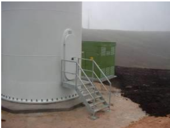
Access to the turbines for maintenance
